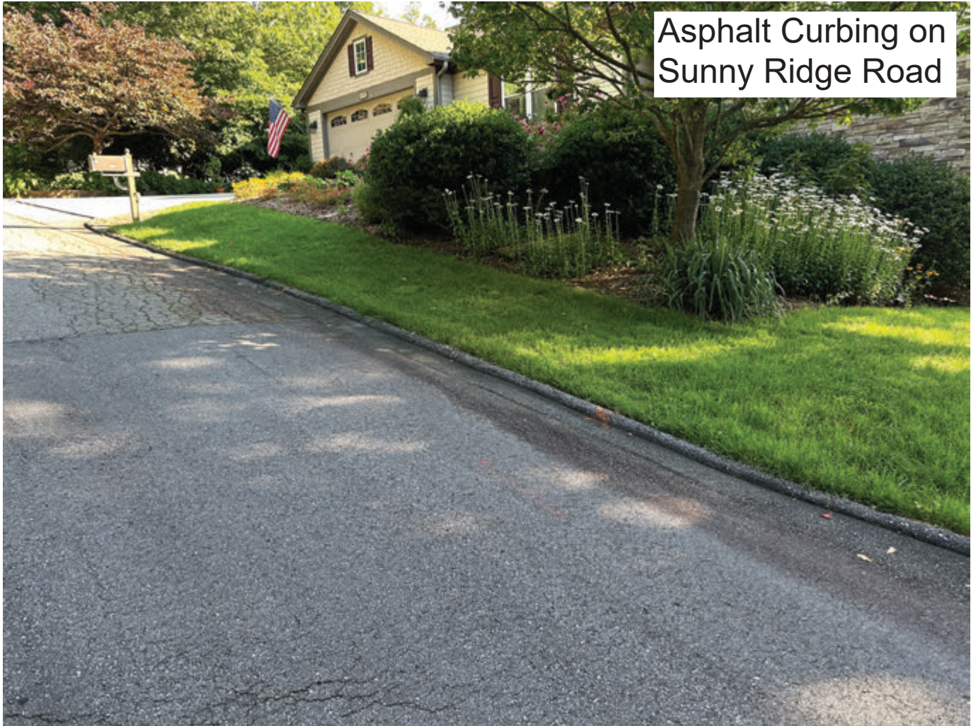
Asphalt Curbing on Sunny Ridge Road
