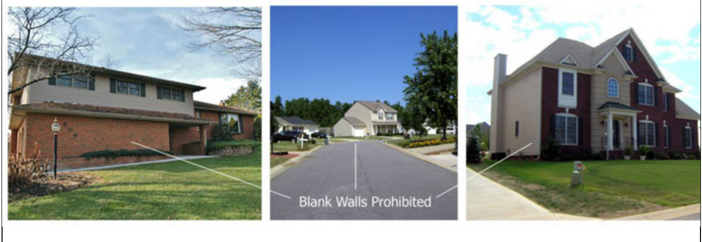
FIGURE 7.1.4:D:4: BUILDING FACADES
