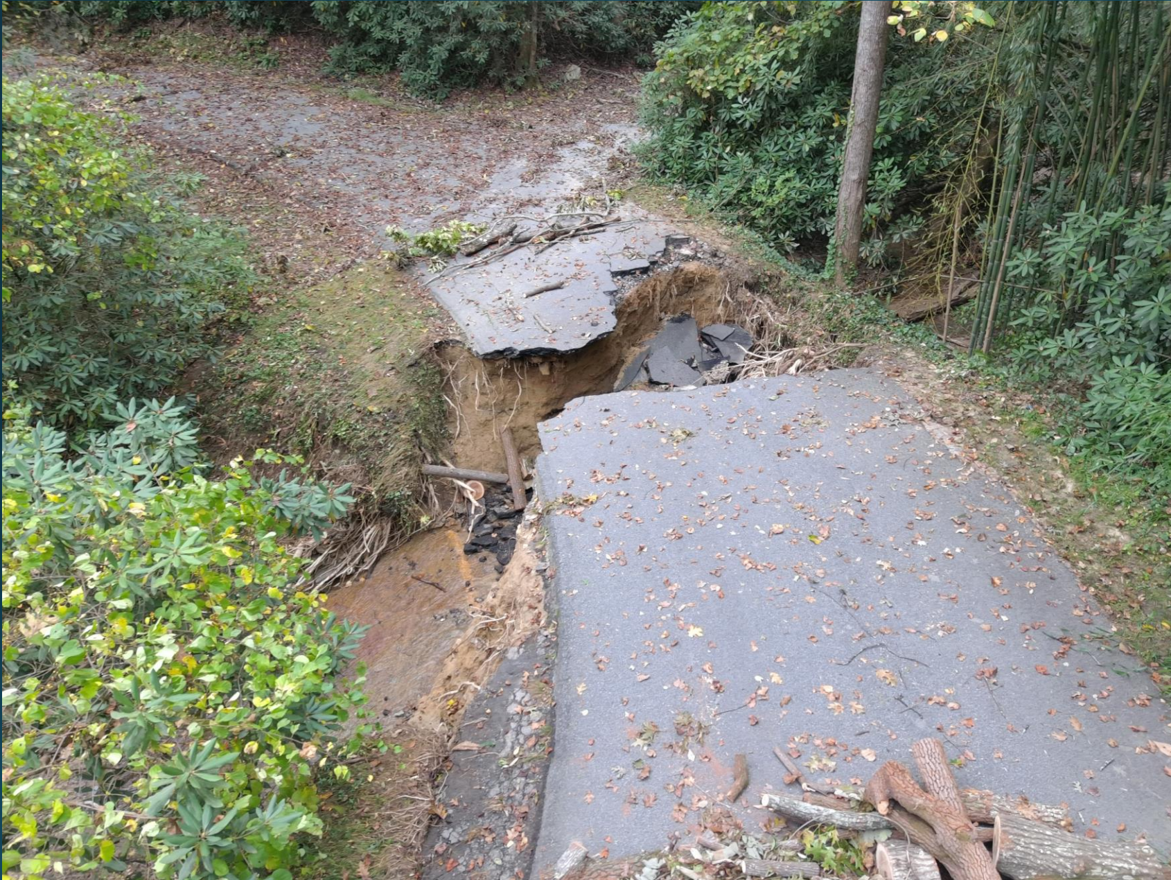
Culvert - Ransier Drive
