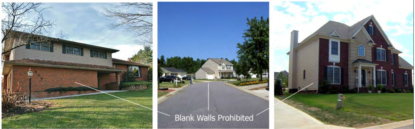
FIGURE 7.1.4:D:4: BUILDING FACADES
