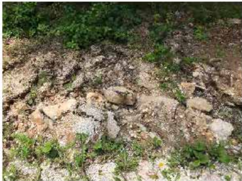
Image 8- Sedimentation on southern slope below the driveway.
