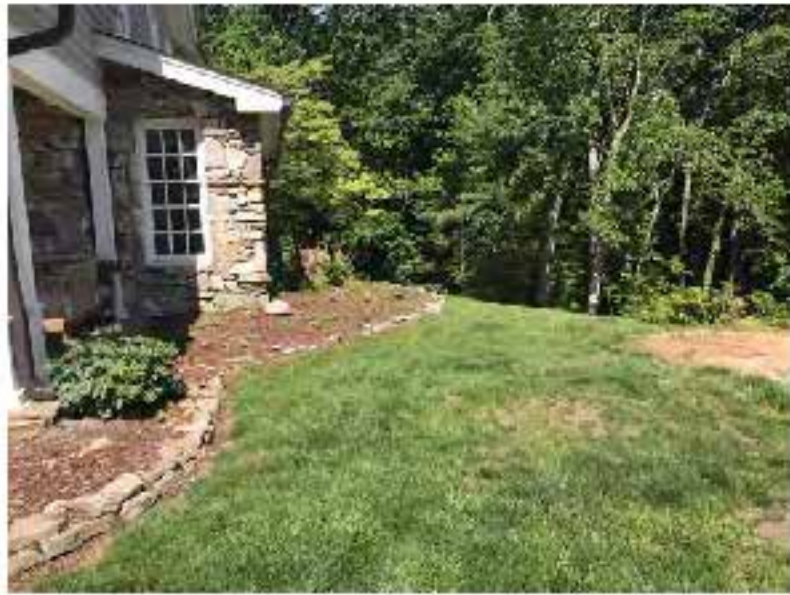
Image 2- Proposed area of disturbance on the northern side of the home. Proposed work here includes addition of patio, steps, walkway, and retaining wall.
