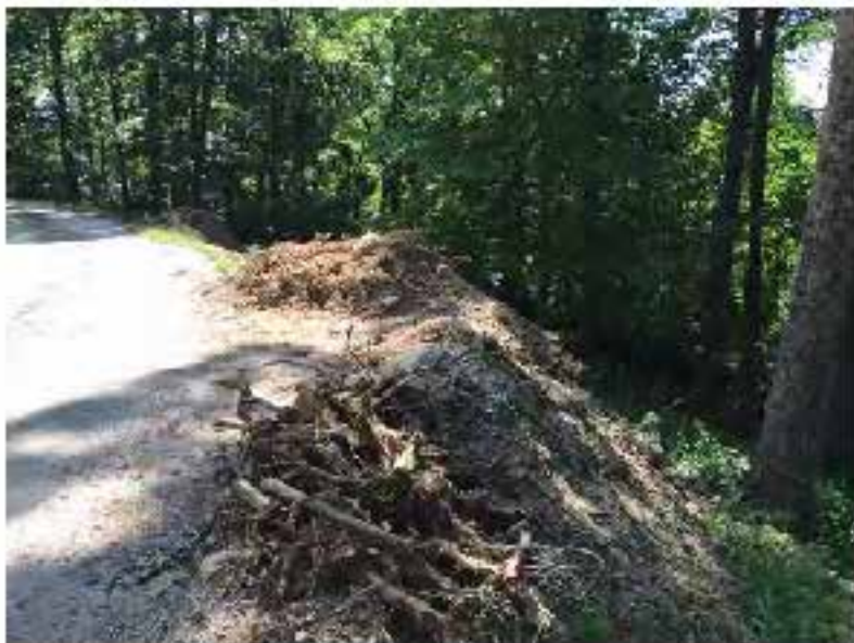
Image 7- View of unstable temporary soil stockpiles along the driveway, below the home, and above the southern slope.
