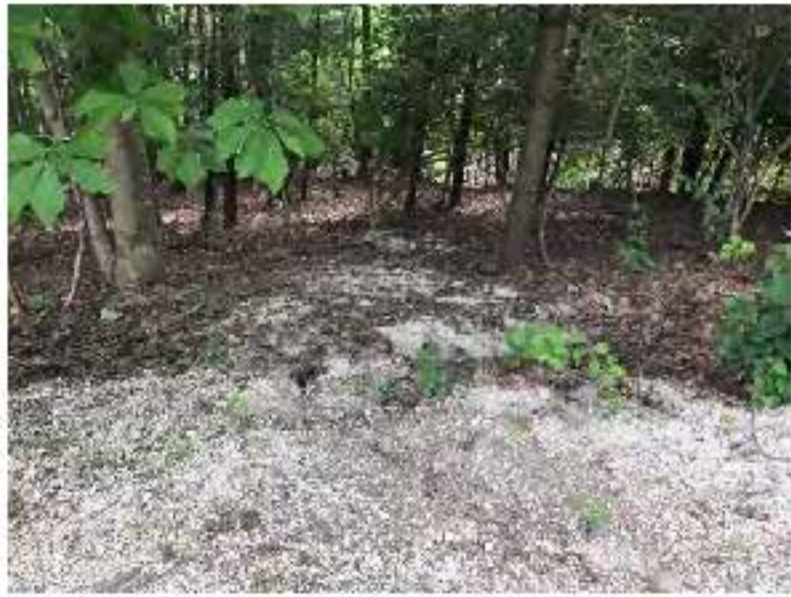
Image 17- Driveway gravel sedimentation downhill from steep driveway. View of adjoining condominium to the east is in the background.
