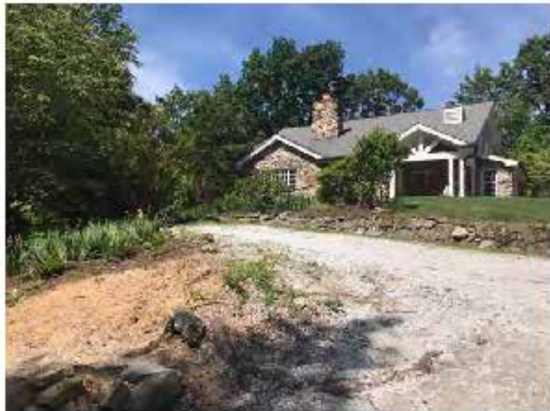
Image 4- Proposed area of disturbance on the east side of the home. Proposed work here includes new parking spaces, steps, and retaining wall.
